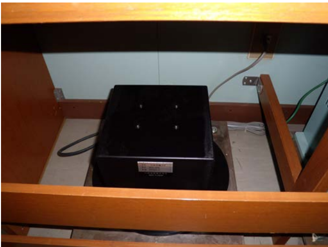
Figure 6-8-3 Attitude sensor (Gravity meter room)
