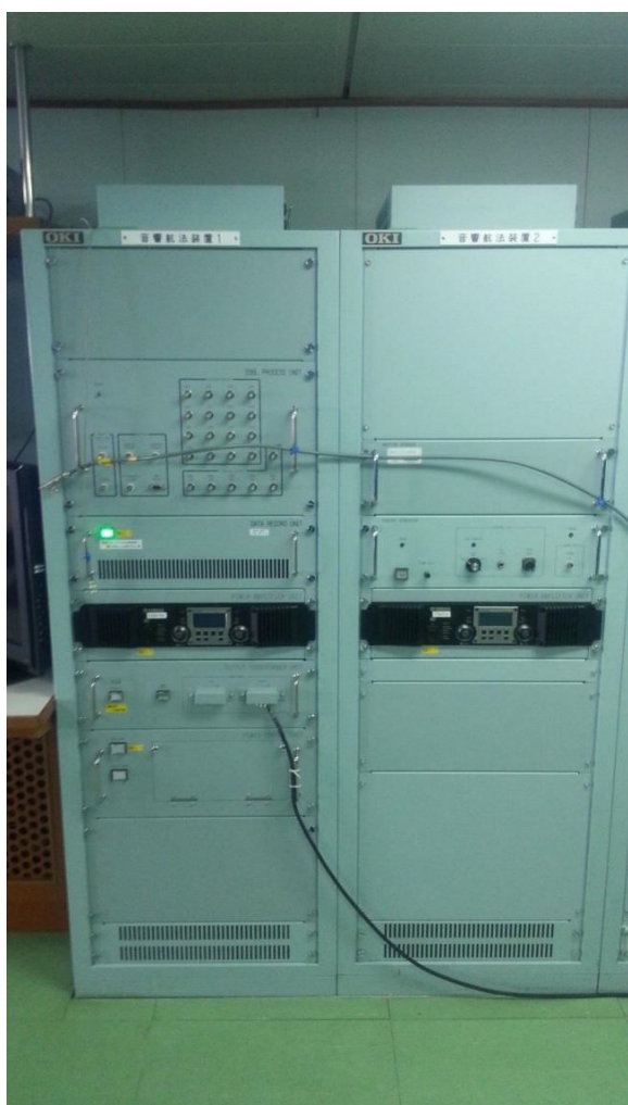
Figure 6-5-1 The ANS is located in the conductor room on the bridge deck.
