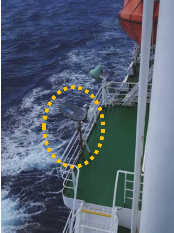
Figure 2.11.2-1: Photo of the antenna unit of the MRR
