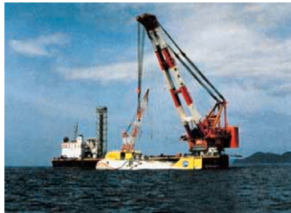
写真 8 係留設置工事 Photo 8 Mooring work of prototype
