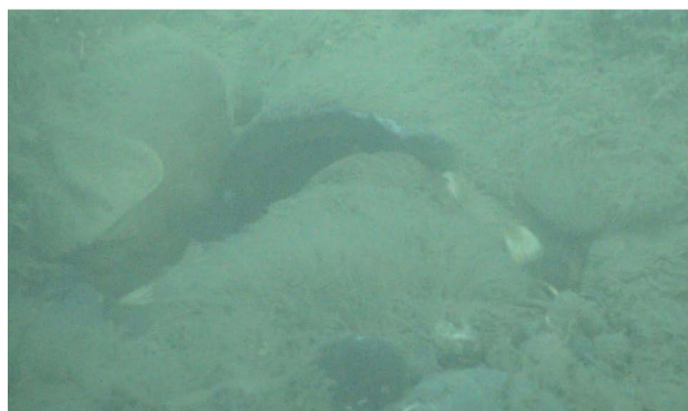
Close-up of the intake
