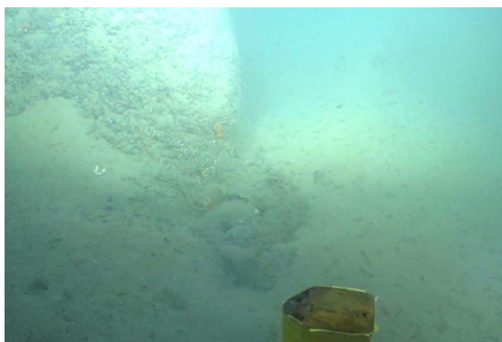
Deep-sea water intake
