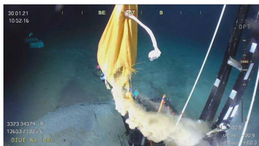
Fig.3-6.3 Backfilling trial
