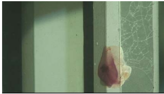
Fig.3-4-3-7 Photo of the junction unit - 5
