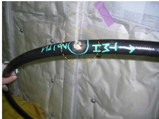
Fig. 3: Air hose failure ahead of the airguns
