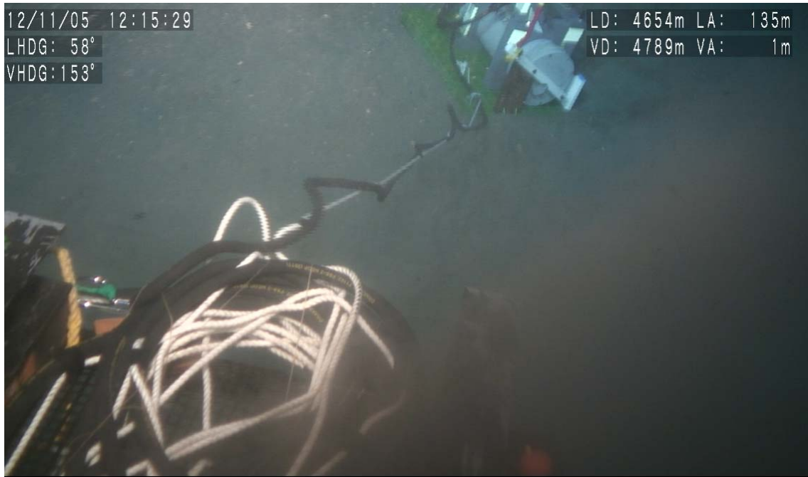
Installation of the Extension Module during dive 583. 2: Extending the cable
