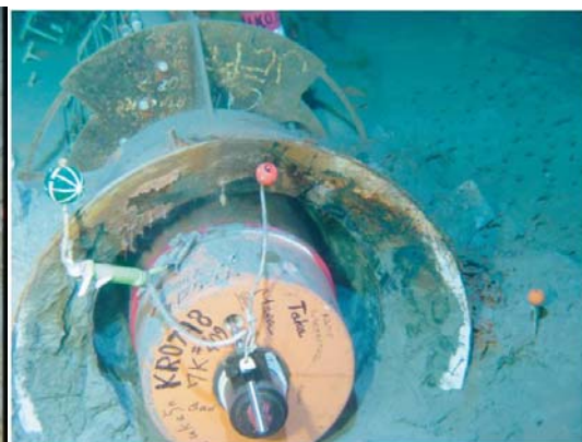
2007 First bridge plug installed
