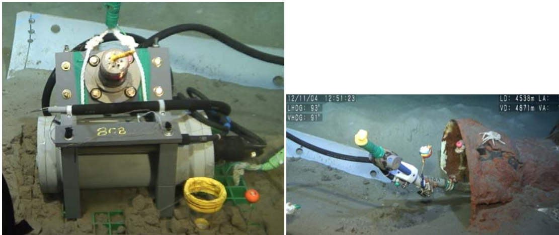
The new pressure data logger installed at ACORK 808I.
