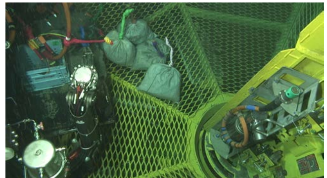
Fig.2-2 Sandbags were put on temporary
