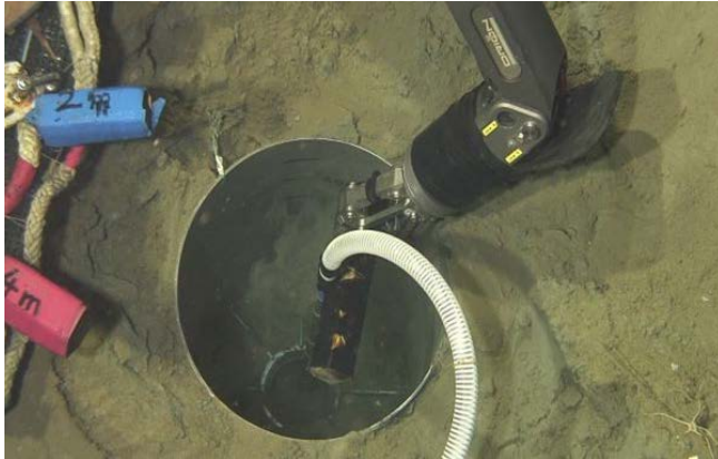
Photo 3. 1-3 Removal of the sediment inside the casing
