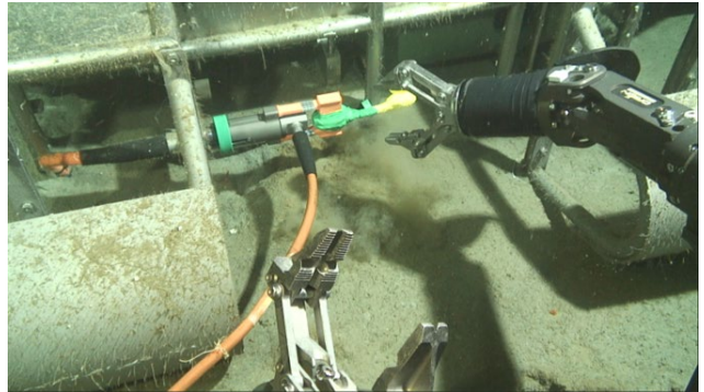
Photo 3.3-2 NODE A040 connected to TU-1A
