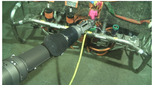
Photo 3.1-4 1A-3 disconnection from Port 3
