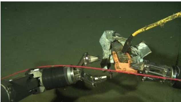
Photo 4.5-3 Pass the connector beneath the new extension cable (red cable).
