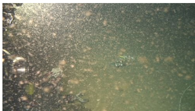
Photo 4.1-2 Junction Box seen through large snowflakes.
