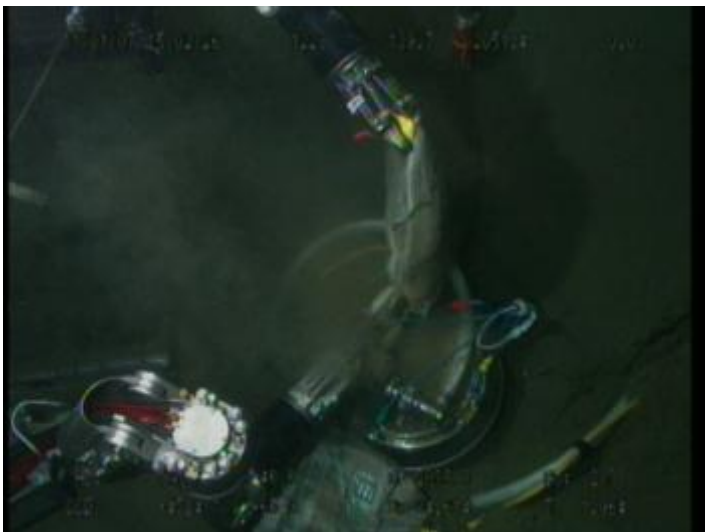
Photo 29 Burial hole back filling by sand bags
