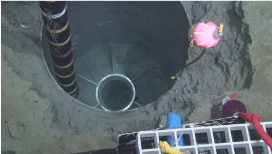
Photo 33 Burial hole conditioning operation at the B-5 site candidate
