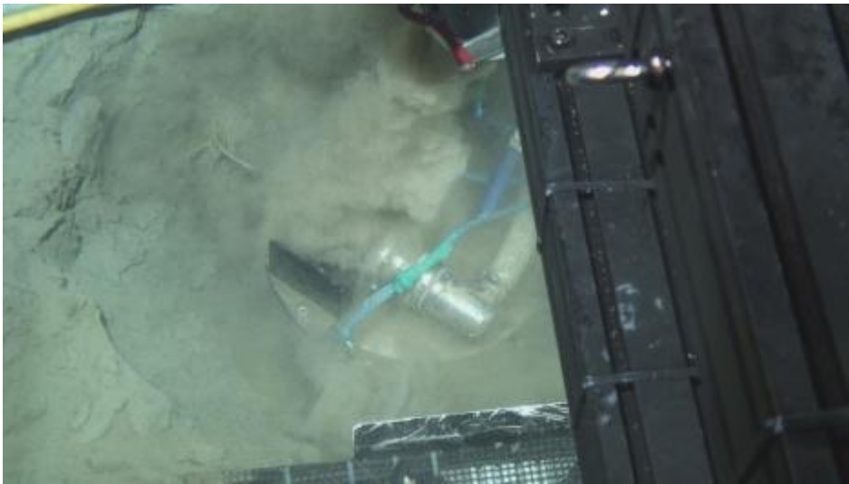
Photo 37 Backfilling burial hole by “sand feeder”
