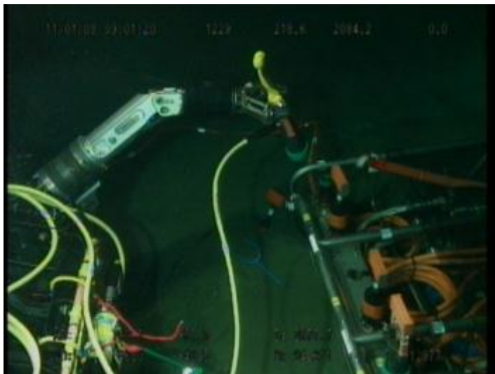
Photo 30 Connection of the cable end to the science node D port No.7
