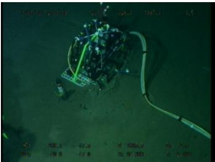
Photo 36 Deployment of pressure sensing system.
