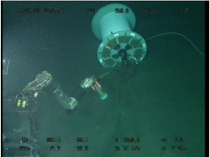
Photo 16 Cable bobbin deployed near the node B
