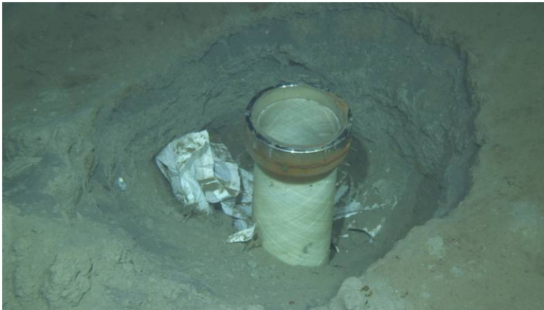
Fig. 3.3 Bottom casing at E-20b'
