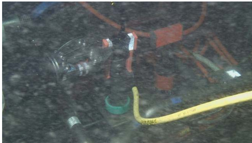
Fig3.33 The extension cable was connected to port No.2
