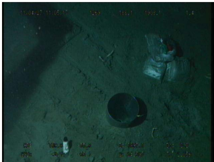
Fig. 3.14 Casing and sand bags
