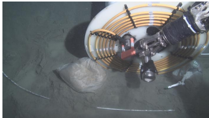
Fig. 3.13 The sand bags to prevent the slippage and rolling (C-10)
