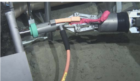
(c) Connection with the terminal
