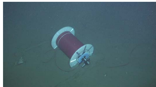
(b) Cable bobbin installed near the casing 2A-3b
