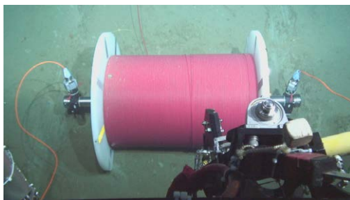
(a) Loading up operation of the cable bobbin.
