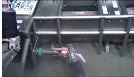
(b) Connecting a loopback connector to TU 2D
