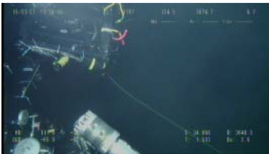
(c) Cable laying operation
