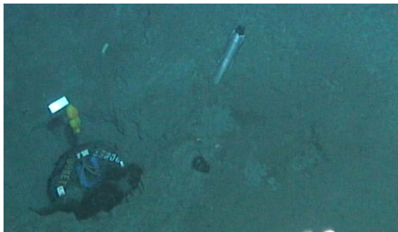
(a) Caisson and a cover plate before the installation
