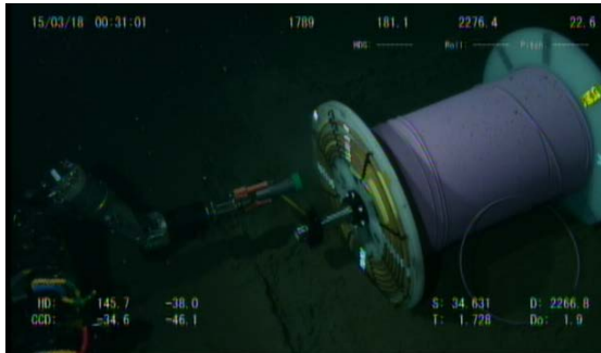
(c) Cable bobbin with cable on the seafloor
