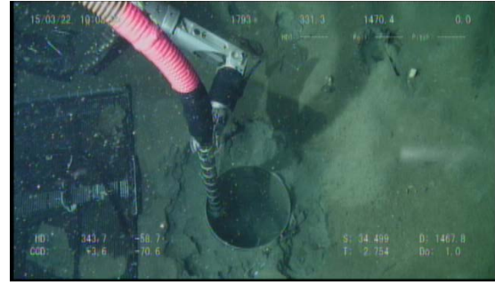
(b) Cleaning inside the caisson
