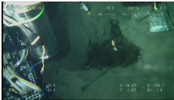
(a) Caisson and a cover plate with seaweed before the installation
