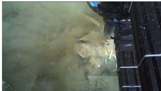
(b) Backfilling the seismometer
