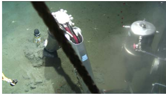
(b) Oil leak from the compensator
