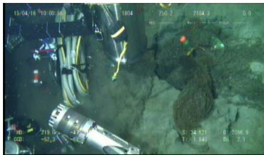
(a) The lid on the caisson was covered with seaweed
