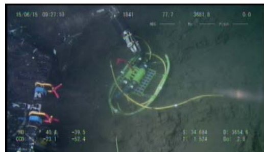
(b) Installation of the junction box
