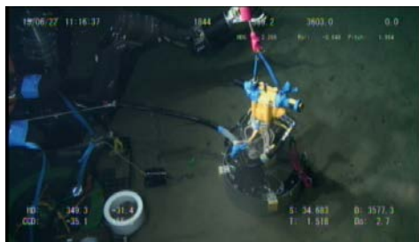
(a) Caisson installation operation
