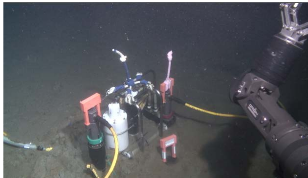
(e) The cable from “Node 2F” was connected to observatory “2F-23”
