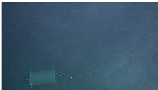
(c) The cable bobbin placed on the seafloor
