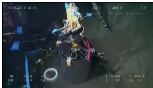
(a) Caisson installation operation
