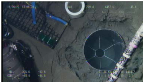
(c) After cleaning inside the caisson
