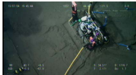
(d) After connection with the battery equipment
