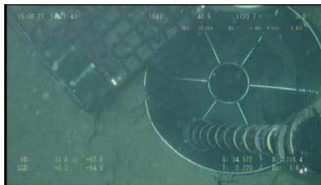
(c) After cleaning inside the caisson
