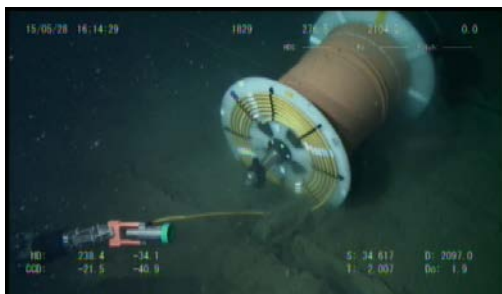
(c) Placing the cable bobbin on the seafloor
