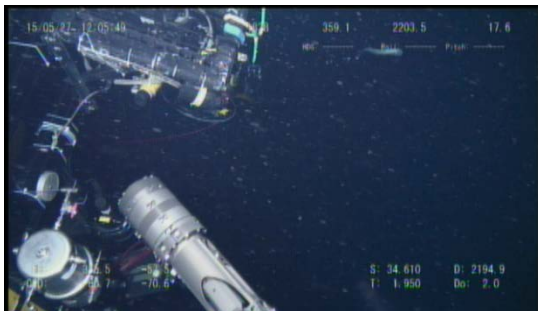
(c) Cable laying Operation
