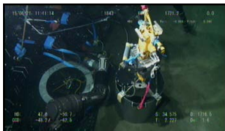
(a) Caisson installation operation
