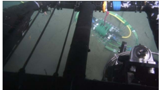
(b) Installation of the junction box
