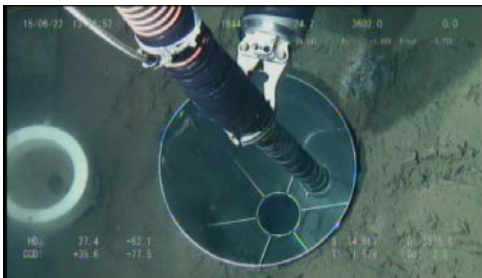
(c) Inside the caisson after cleaning
