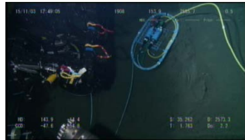
(b) Placing the junction box on the seafloor
