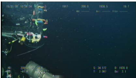
(c) Cable laying operation
