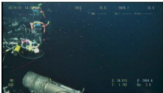
(c) Cable laying Operation
