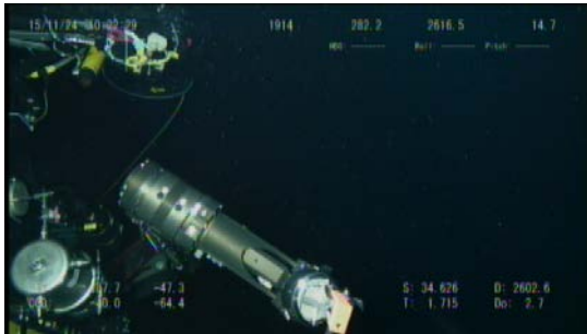
(c) Cable laying Operation
