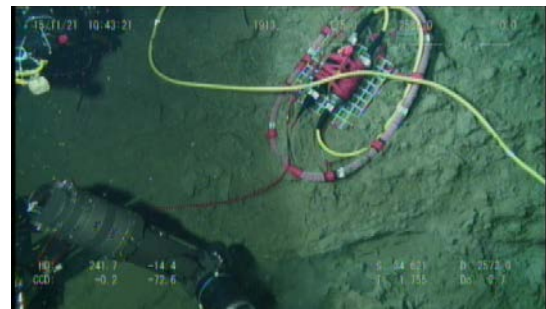
(b) Installation of the junction box
