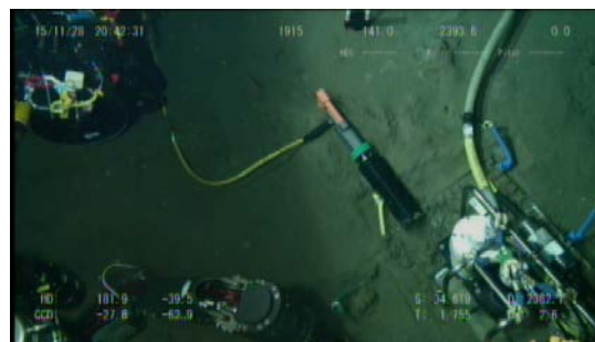
(e) The cable from Node 2F was connected to observatory 2F-24
