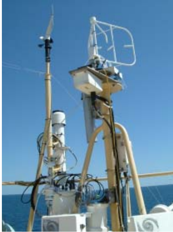
Fig.7.9-1 Installation of the turbulence measurements sensors at the top of the foremast.
