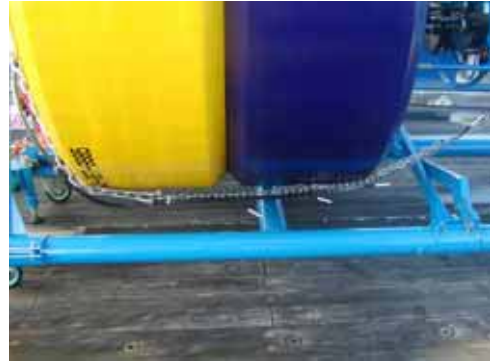
Fig. 5.14.3-2 The thermistors (white bar connected to black signal cable) installed along the stainless chain.
