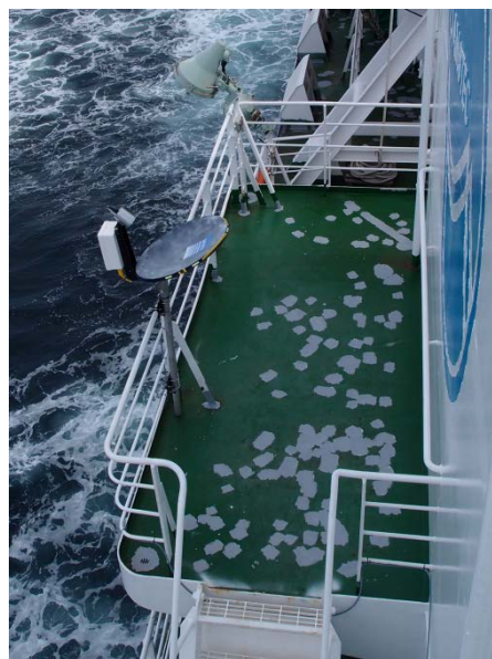
Photo 8.1.5-2: The micro rain radar, installed on the starboard side of the anti-rolling tank.
