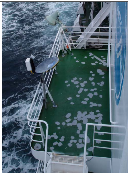
Fig. 6.8-2: The micro rain radar, installed on the starboard side of the anti-rolling tank.
