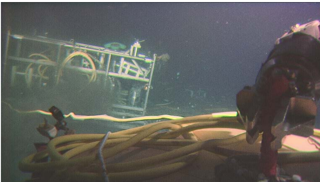
Fig. 3. Cable extension from Hatsushima observatory to the lander. The extension cable was mounted on a special cable rack in the payload developed by “Hyperdolphin team”.
