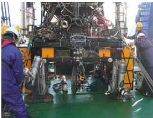
Photo 1 Cable Laying System
