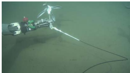
Photo 2 Cable End Anchor
