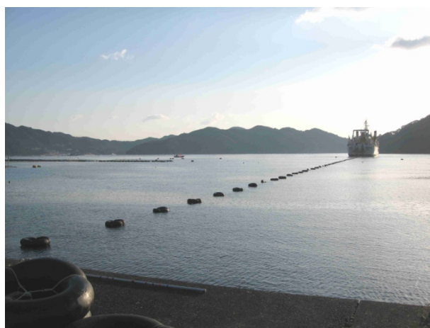
Photo 2 Landing a cable end at Kata-bay, Furue-cho Owase
