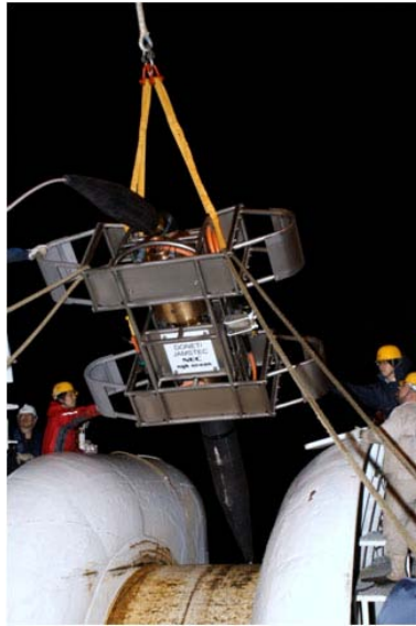
Photo 3 Installation of Termination Unit
