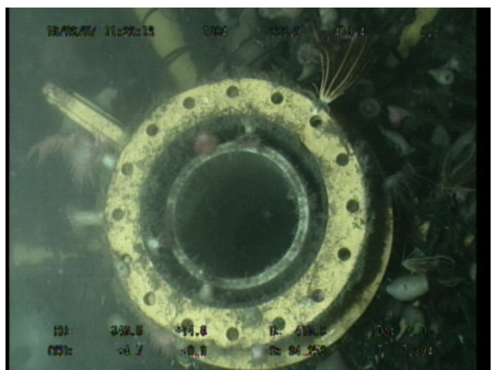
Photo 11 Close up of water intake
