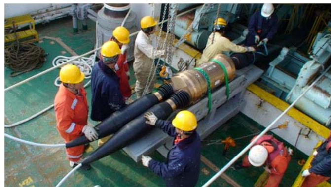
Photo 5 Branching Unit on Deck
