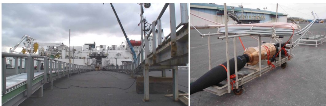
Photo 1 Loading of DONET backbone cable system
