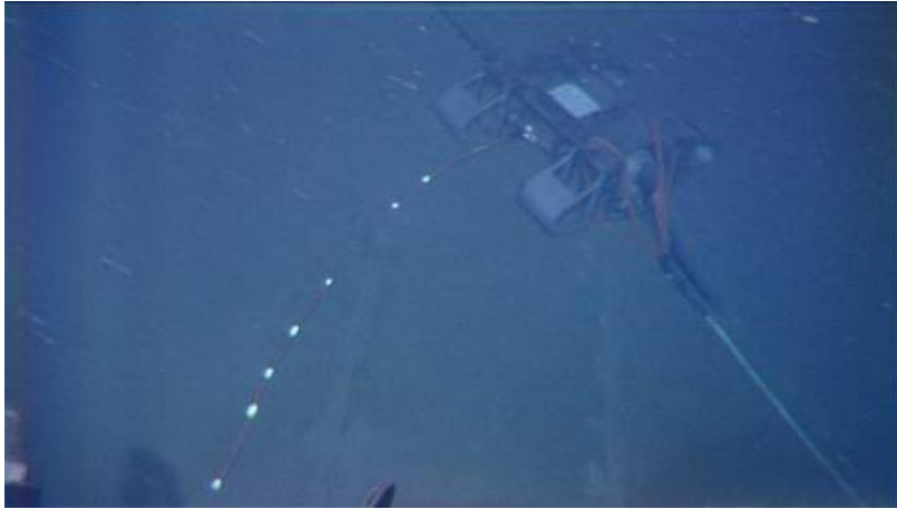
Photo 29 Interconnect cable on seafloor near TU (TU-D)
