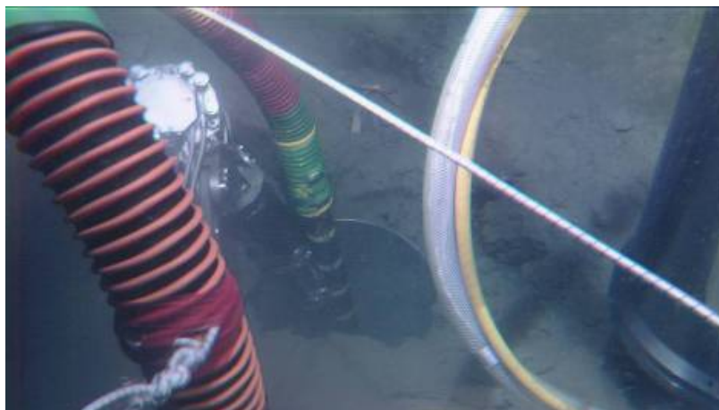
Photo 6 Burial hole conditioning by DOROTHY system
