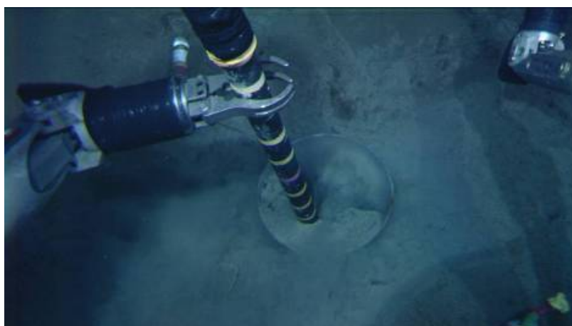
Photo 19 Burial casing conditioning
