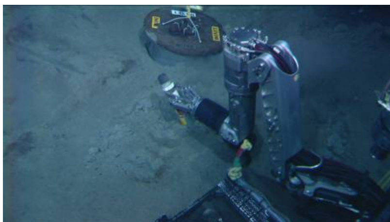
Photo 20 Put a cover on the top of Burial casing
