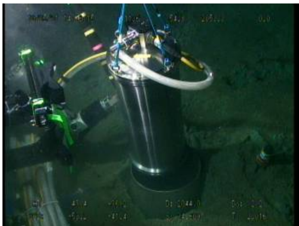
Photo 21 Ground motion sensing system installation at site A-4
