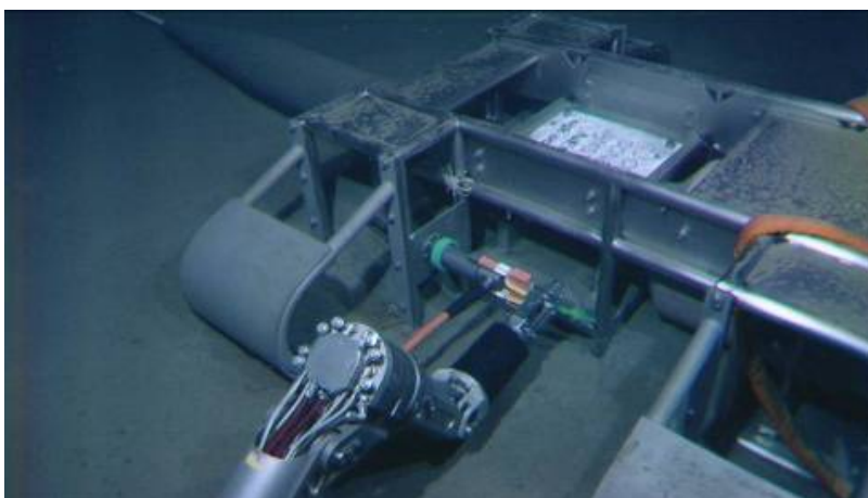
Photo 27 Interconnect cable mating operation to TU-D
