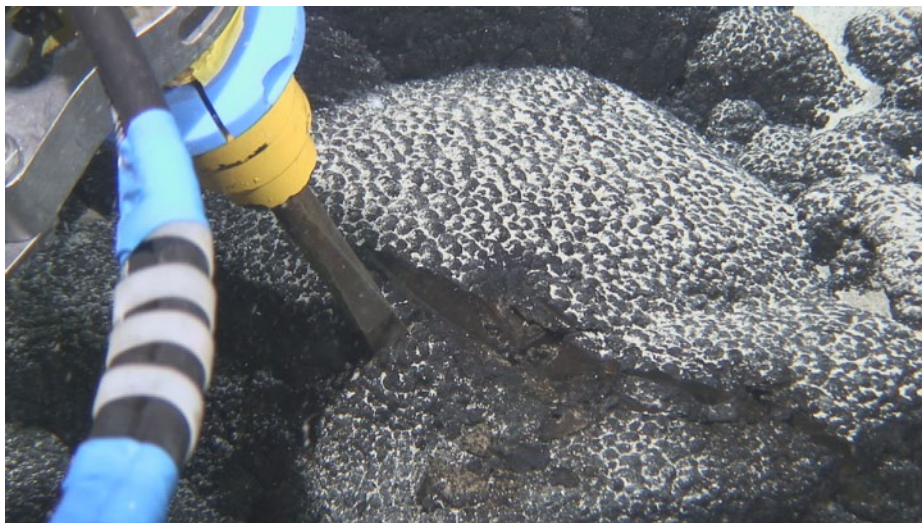
Fig: 11 Rock breaker being used durin drive HPD#1540
