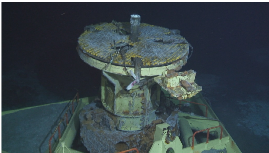
Fig. 2 Corrosion cap on the borehole guide base of C0014G (HPD Dive #1591).
