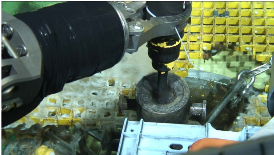
Fig. 3-18 Removing scale within the steel pipe by hydraulic power chisel.
