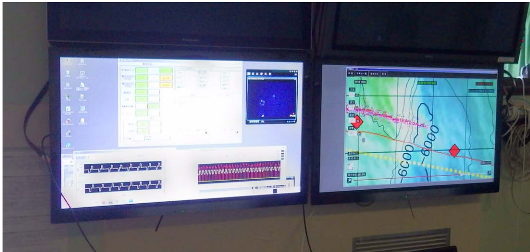
Figure 3.5-1. Onboard monitoring system.
