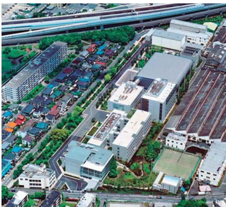
Fig. 8 General view of Yokohama Institute for Earth Sciences
