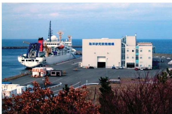
Fig. 3 Observation Equipment and Machinery Maintenance Shop and "MIRAI" in Sekinehama Port.
