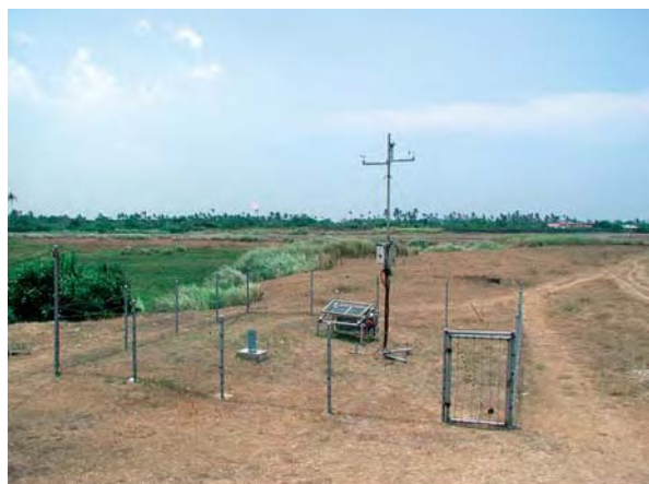
Fig.12 Automatic Weather Station installed in Daet, the Philippines.
