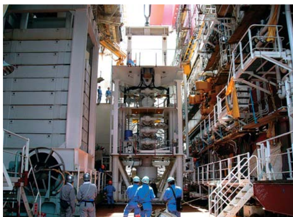
Fig. 2 Installation of Blow-Out Preventer.
