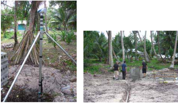
Fig.3 Installation of magnetometer in Majuro (above). Construction of installation site for broadband seismometer in Majuro (bottom).
