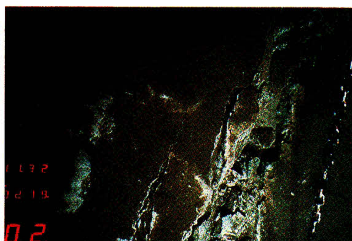
写真10 測線C-3 2 (11時32分02秒) 新しい地割れ [縁が鋭く表層堆積物を切っている] C-3 2 (11:32:02) New cracks. Edges of cracks are sharp and cracks are not filled with sediments.
