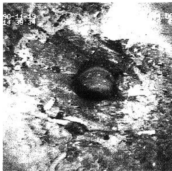
写真9 掘削穴 Photo.9 Drilled Hole
