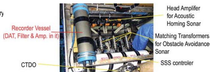
Photo 6 Vessels below Point C
